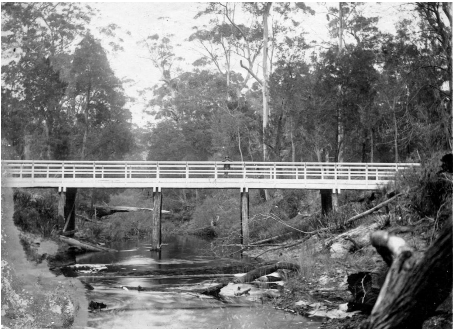
Harry Parker on a refurbished Kent River bridge in the 1950 -1960's - no doubt remembering how he worked on the building of the original bridge. (Picture courtesy Don Burton)
